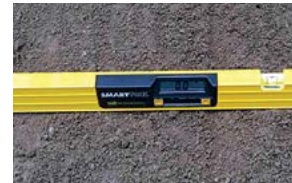
Laser control helps maintain the perfect grade
